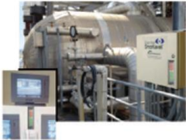
Eye-Hye® SmartLevel™ Local and Remote Indicators
