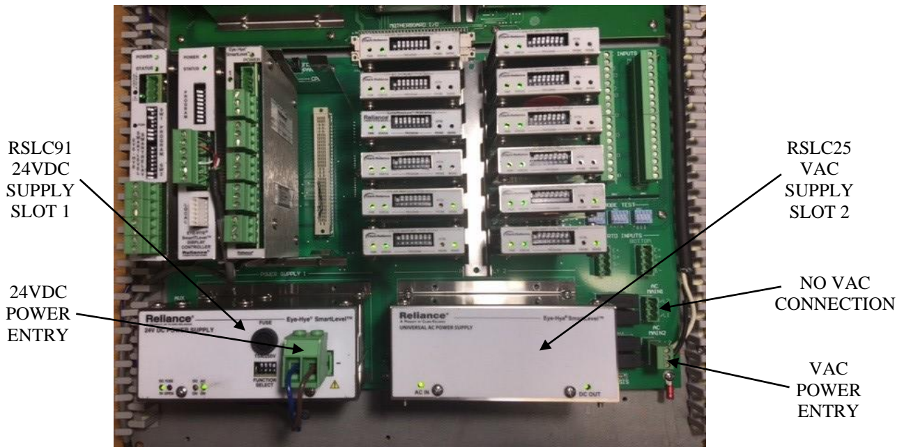
FIGURE 6 – Both 24VDC RSLC91 & AC RSC25 Installed
