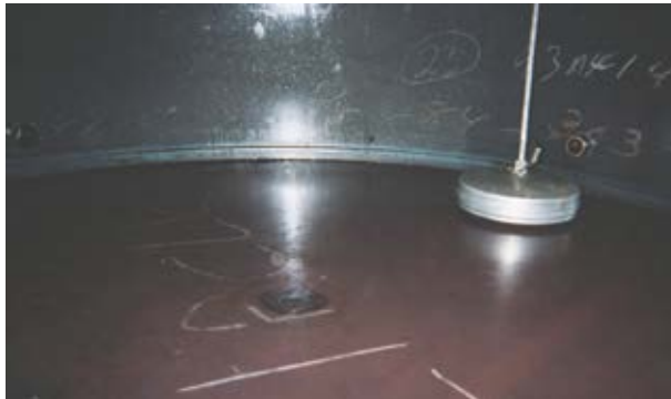
Confined space entry reservoir after cleaning
