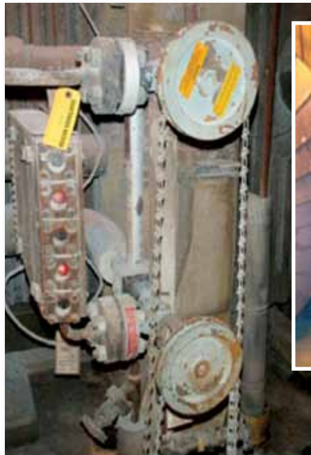
PHOTO A (left): water gauge glass in disrepair. PHOTO B (above): code-compliant water gauge glass.
