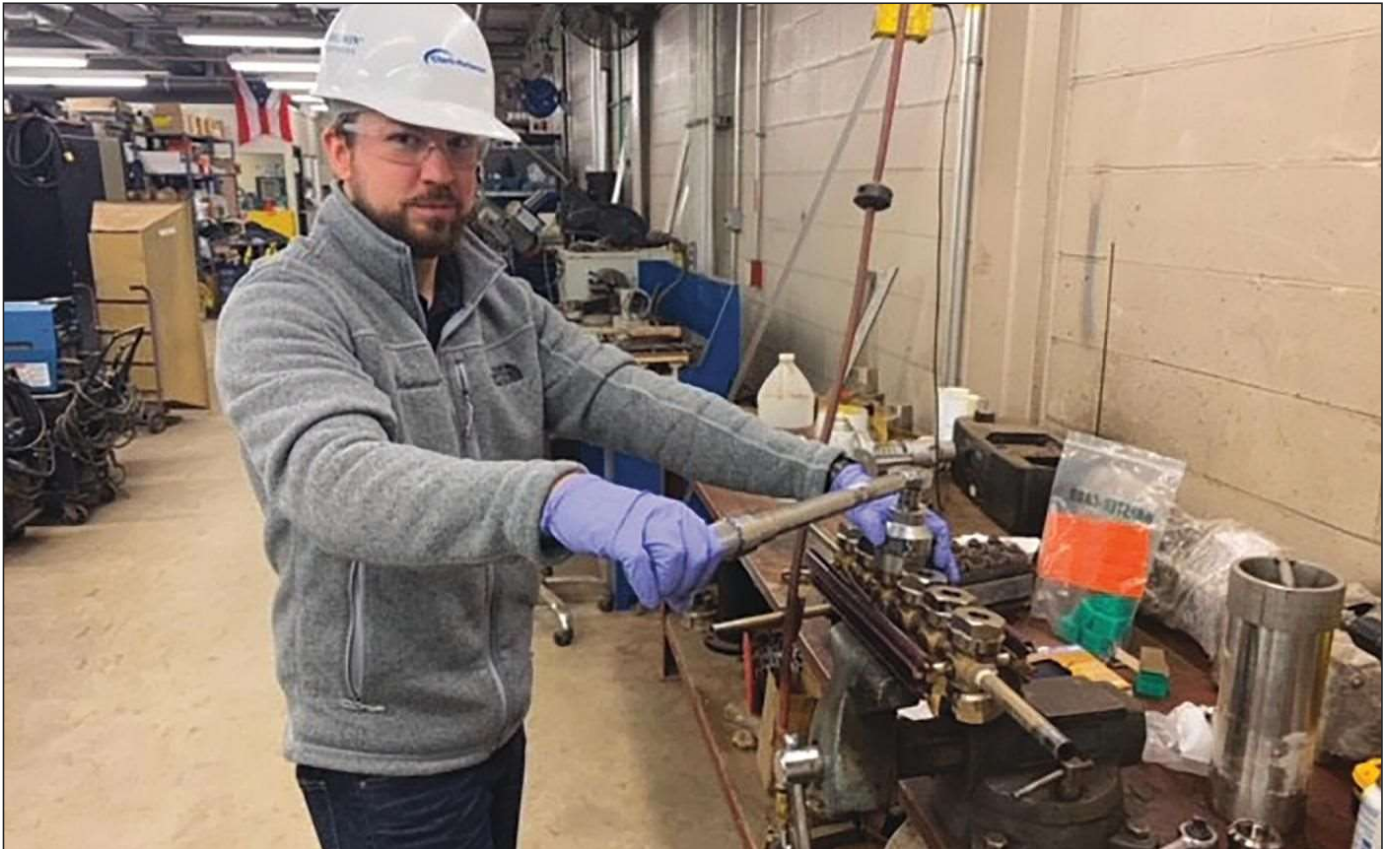
Figure 1: Servicing a water gage glass with a calibrated torque wrench.
