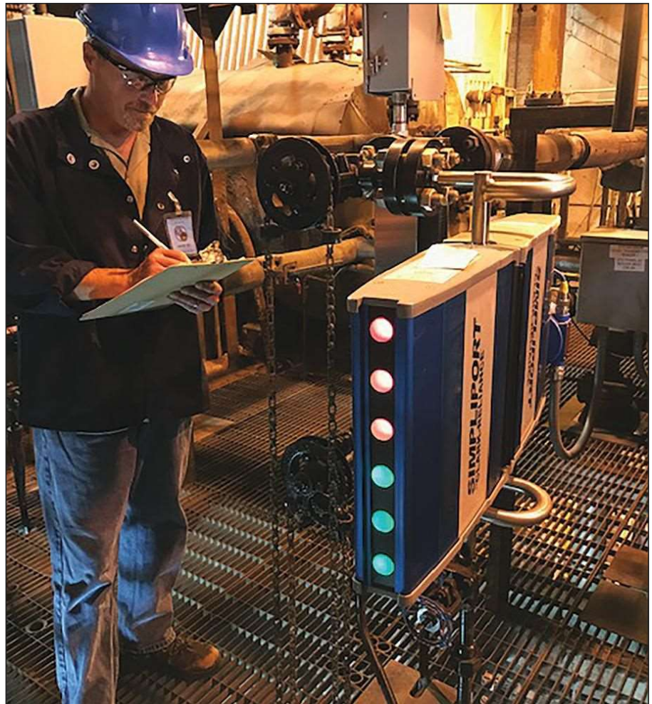
Figure 2. Inspecting water-level instrumentation.
