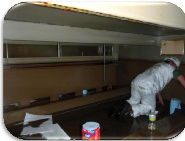
Confined Space Entry Reservoir Cleaning
