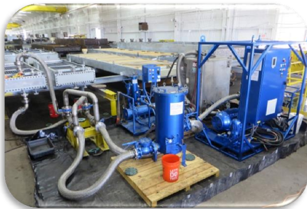
High Velocity Oil Flush of Cooler Bundles
