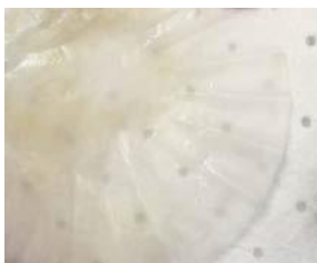
Inspection Screen (After Flush)
