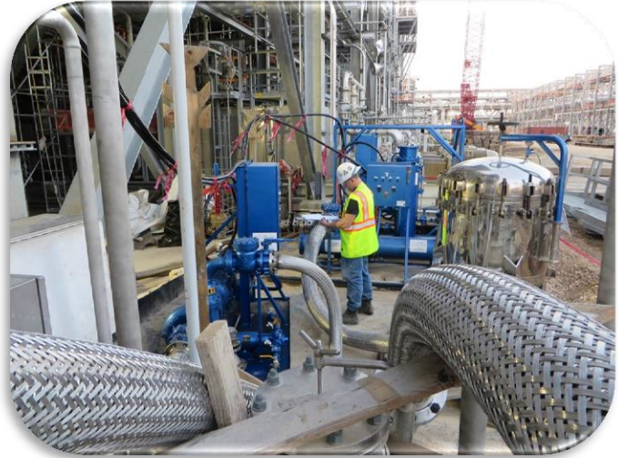
Pre-Commissioning High Velocity Oil Flush at LNG Plant
